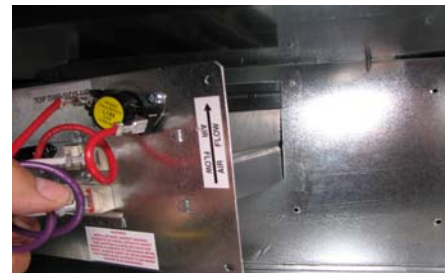
FIG. 1 - Heater assembly insertion.
