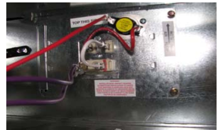
FIG. 2 - Installed heater plate.
