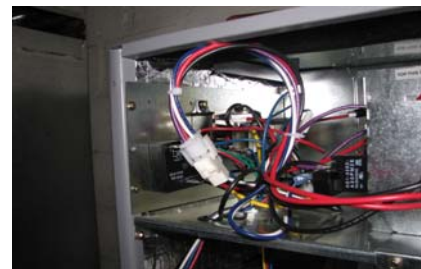
FIG. 3 – Connected (6) pin socket.
