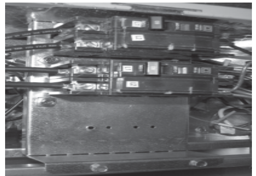
Fig. 3 - Heater bracket installation.
