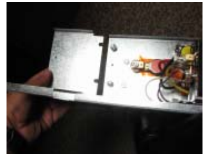
Fig. 1 - Filler plate installation.
