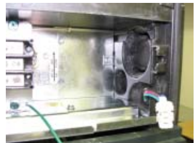
Fig. 2- Installed retainer tab.
