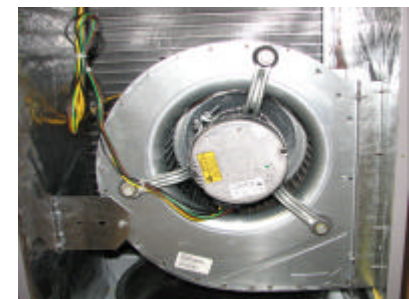
FIG. 2- Blower motor installed
