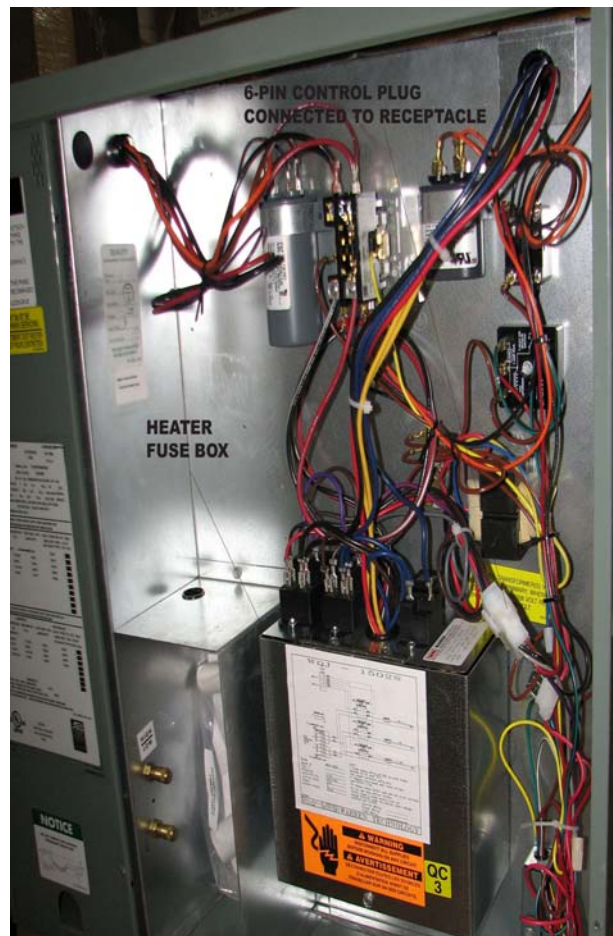
FIG. 3 - Fuse box installation.
