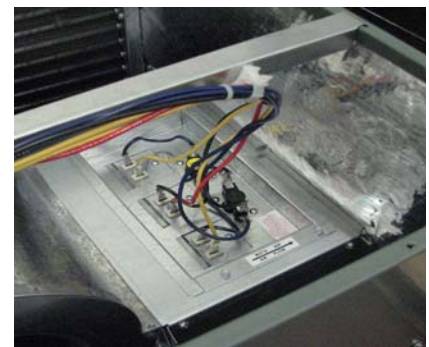
FIG. 2 - Installed element section.
