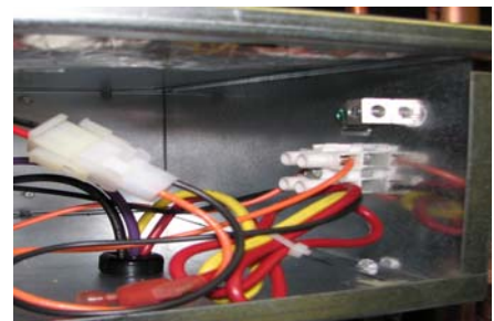
FIG. 3 - Power block with 2-pin connector.
