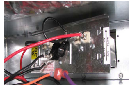
FIG. 1 - Heater assembly insertion.
