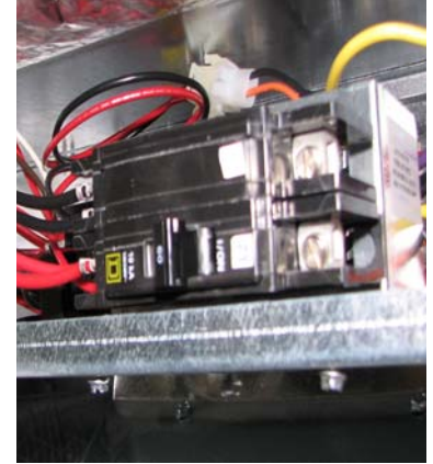
FIG. 4 - Bracket installation.
