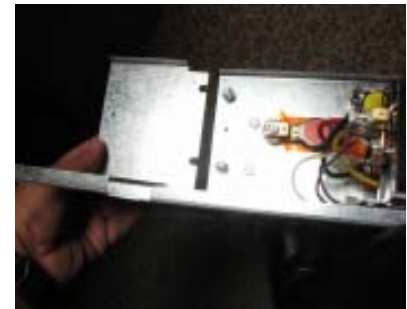
Fig. 1 - Filler plate installation.
