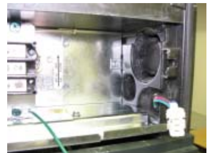
Fig. 2- Installed retainer tab.
