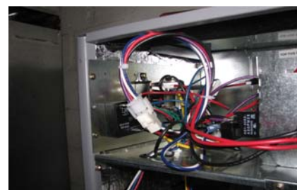
FIG. 3 - Connected (6) pin socket.
