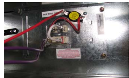
FIG. 2 - Installed heater plate.
