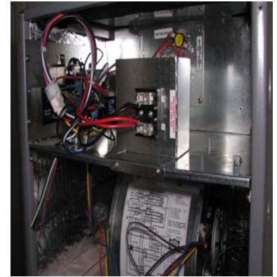
FIG. 4 - Bracket installation.
