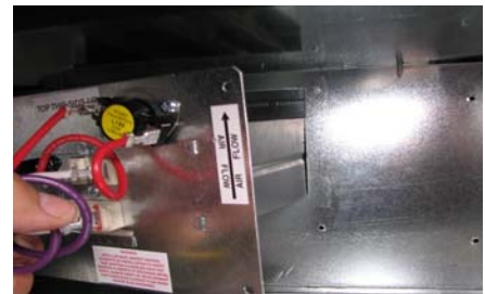
FIG. 1 - Heater assembly insertion.
