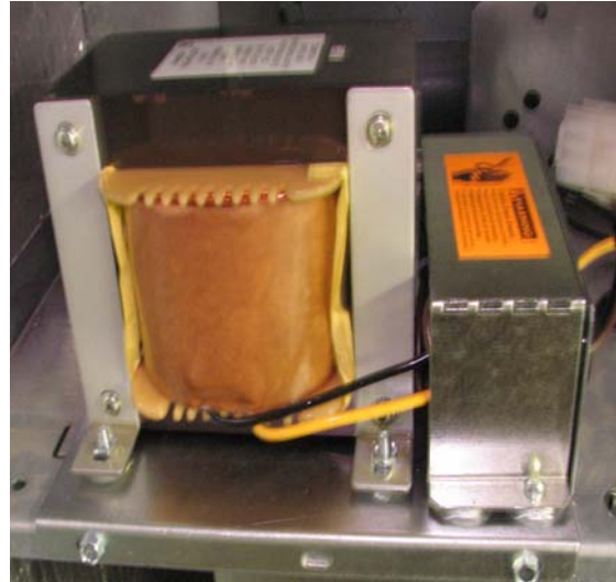
Fig. 1 – WKF autoformer installation.
